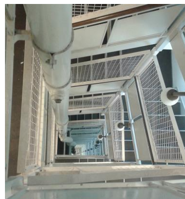
View from the top of the tower staircase
